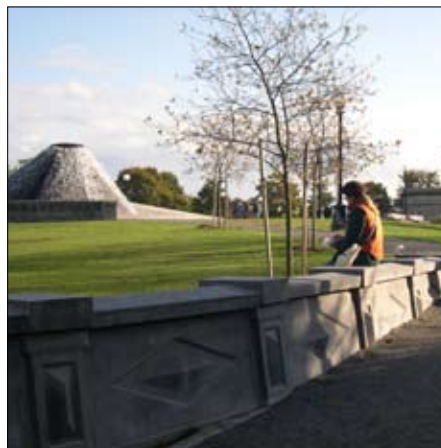
Re-constructed section of the old reservoir walls defines the space and reflects the former design
