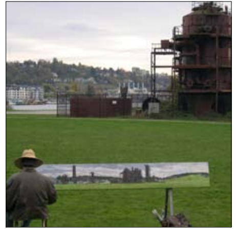
Gas Works Park Seattle, Industrial Heritage preserved as a landmark structure in Rich Haags famous 1980s park
