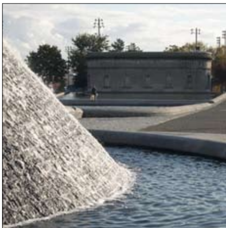
New water feature with pump room in the background
