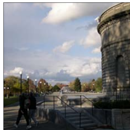
Pump house restored
