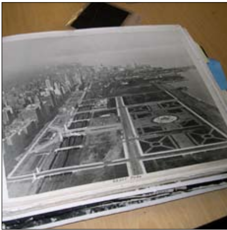
Photos of the initial construction of Grant Park from the Chicago Park District Archives
