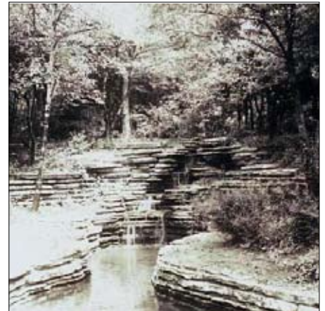
Original construction of stratified rockwork and waterfall
