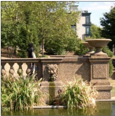
Fountain inset into walls of the grand Cascade, showing fine detail of the exposed aggregate structure
